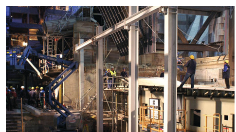
Cooler during erection
