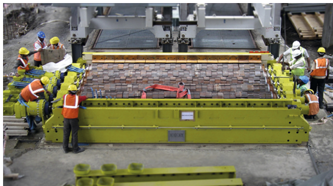
Installation on site
