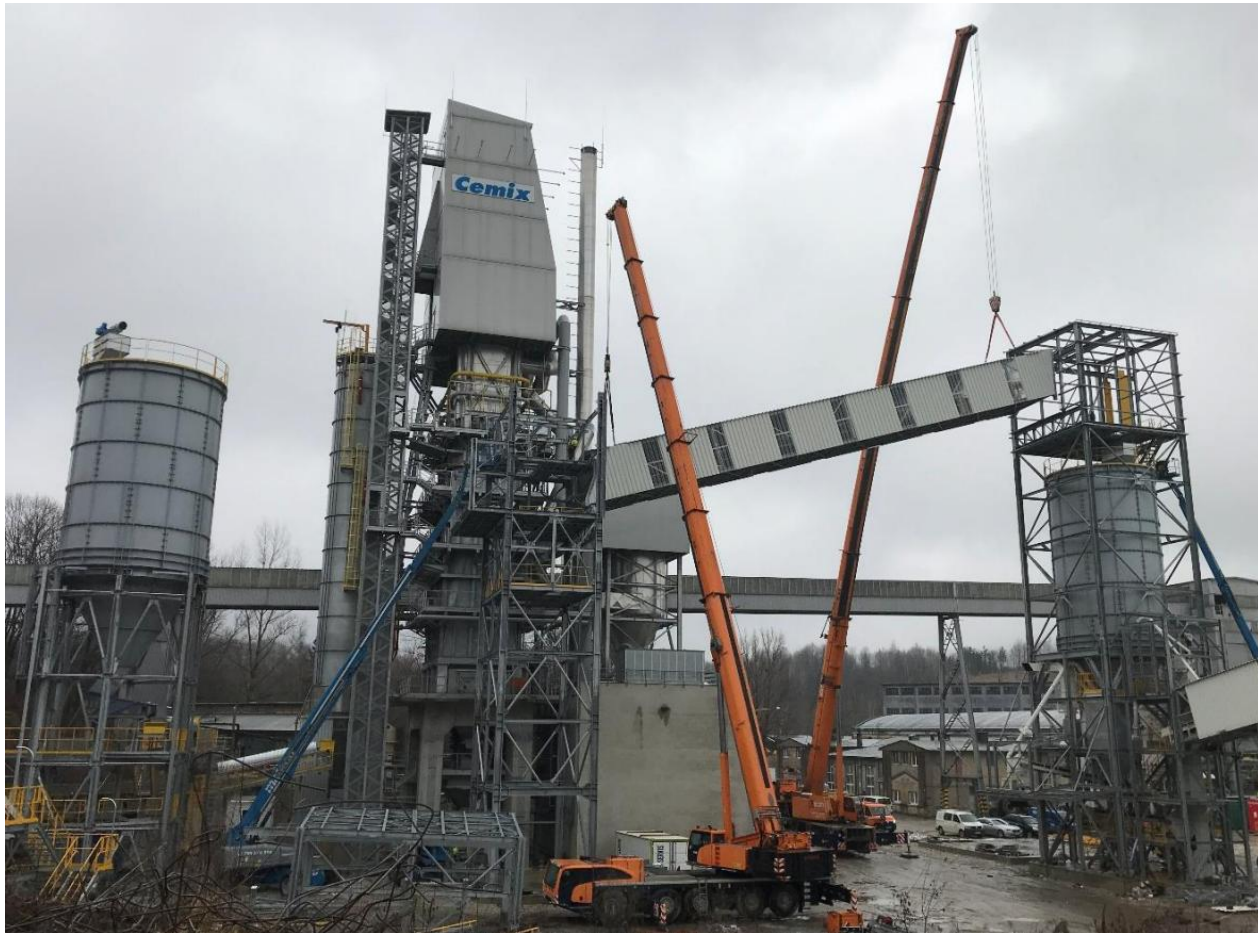
Transport of lime from the shaft kiln to the silo in front of the mill
