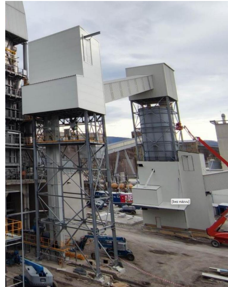
Transport of lime from the shaft kiln to the silo in front of the mill
