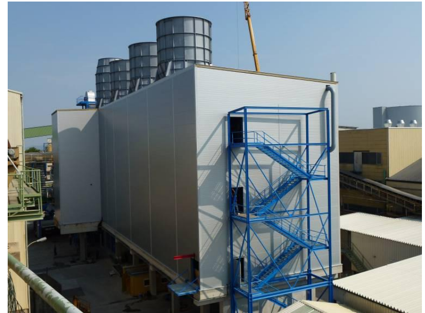
Belt Dryer in Tulln AT, - 45 t/h – 870 m 2 drying of Sugar Beet Pulp
